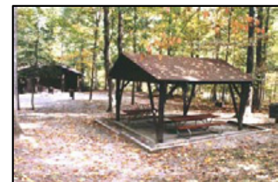
Picnic Pavilion at Locust Shade Park
