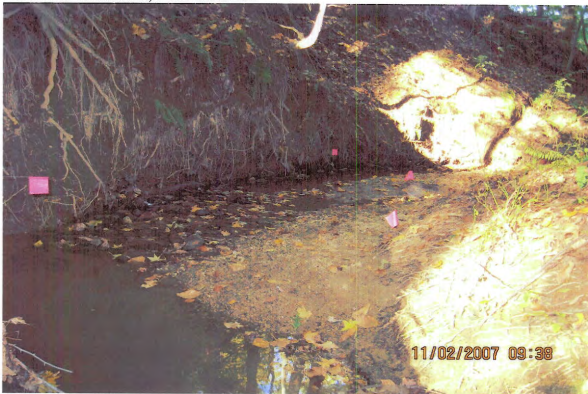
BEFORE - Location to excavate channel bar near right bank and stabilize the left stream bank.
