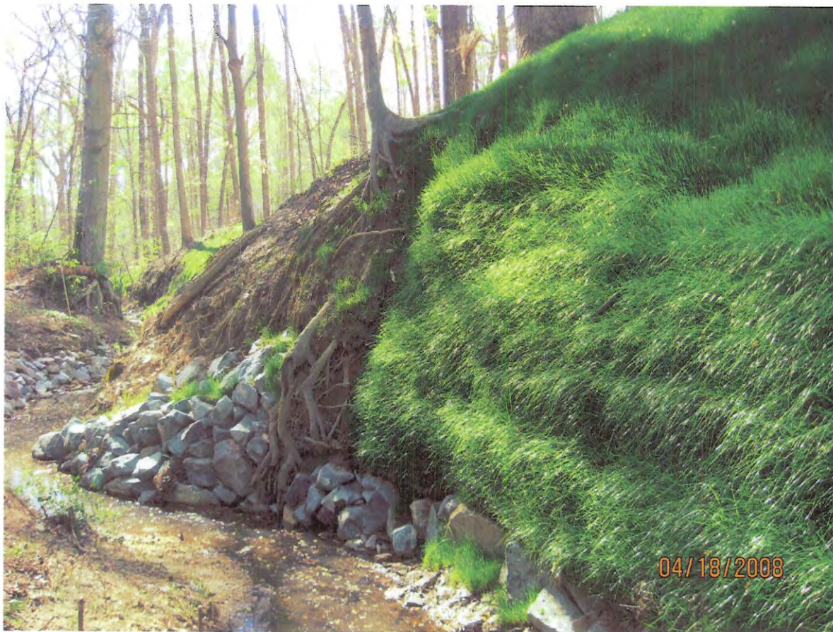
AFTER - Location #7, stabilize bank with toe stone, filtrex sox and backfill.
