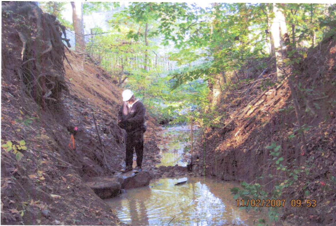
BEFORE - Rock weir #5 under construction.
