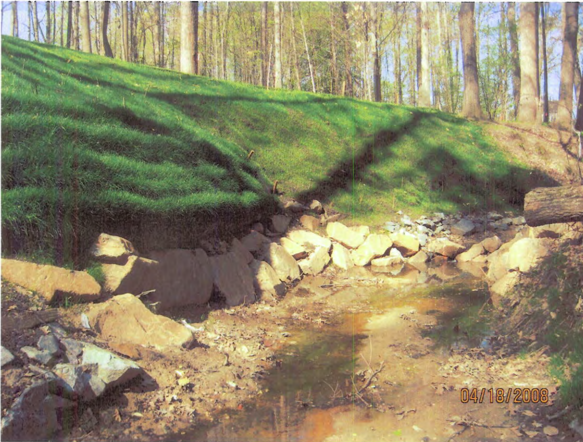
AFTER – filtrex sox supported by rock toe structure and bank stabilization with compost tea.
