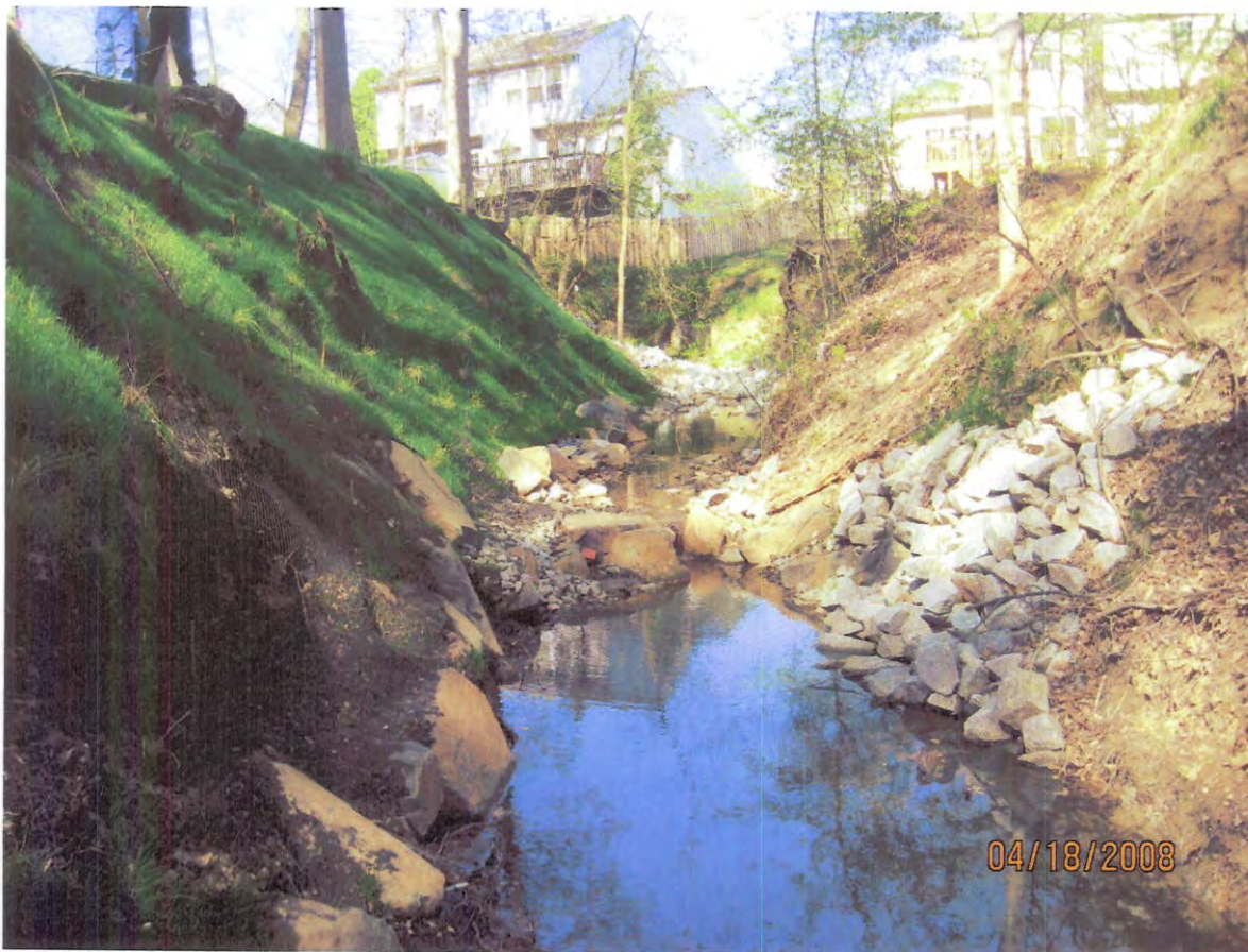
AFTER - rock weir #5.
