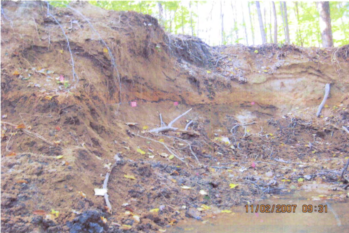
BEFORE – Eroded left stream bank before stabilization.
