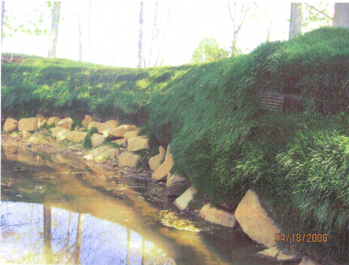
AFTER – above weir #4 continued.
