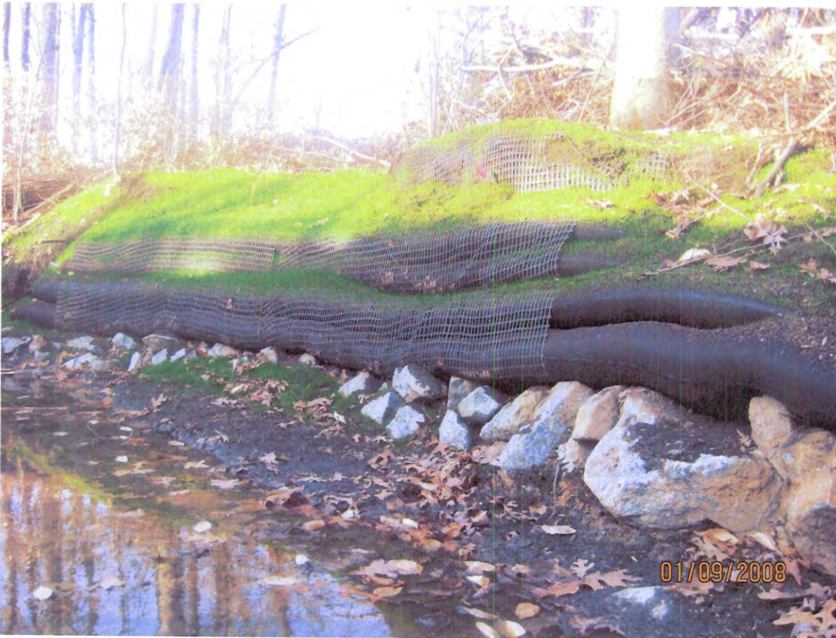
AFTER - rock toe treatment filtrex bank stabilization.
