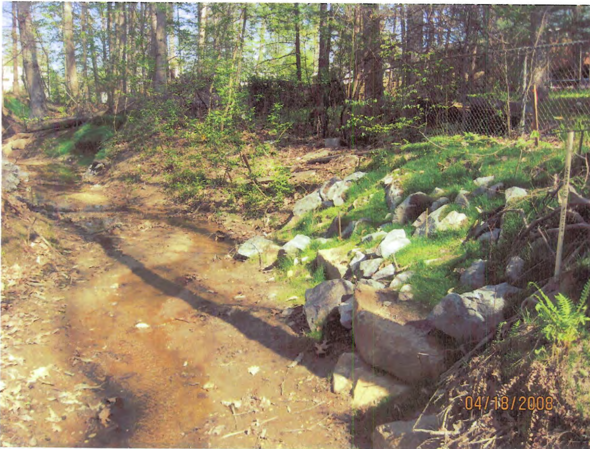
AFTER - Location #4, stone toe and bank stabilization.
