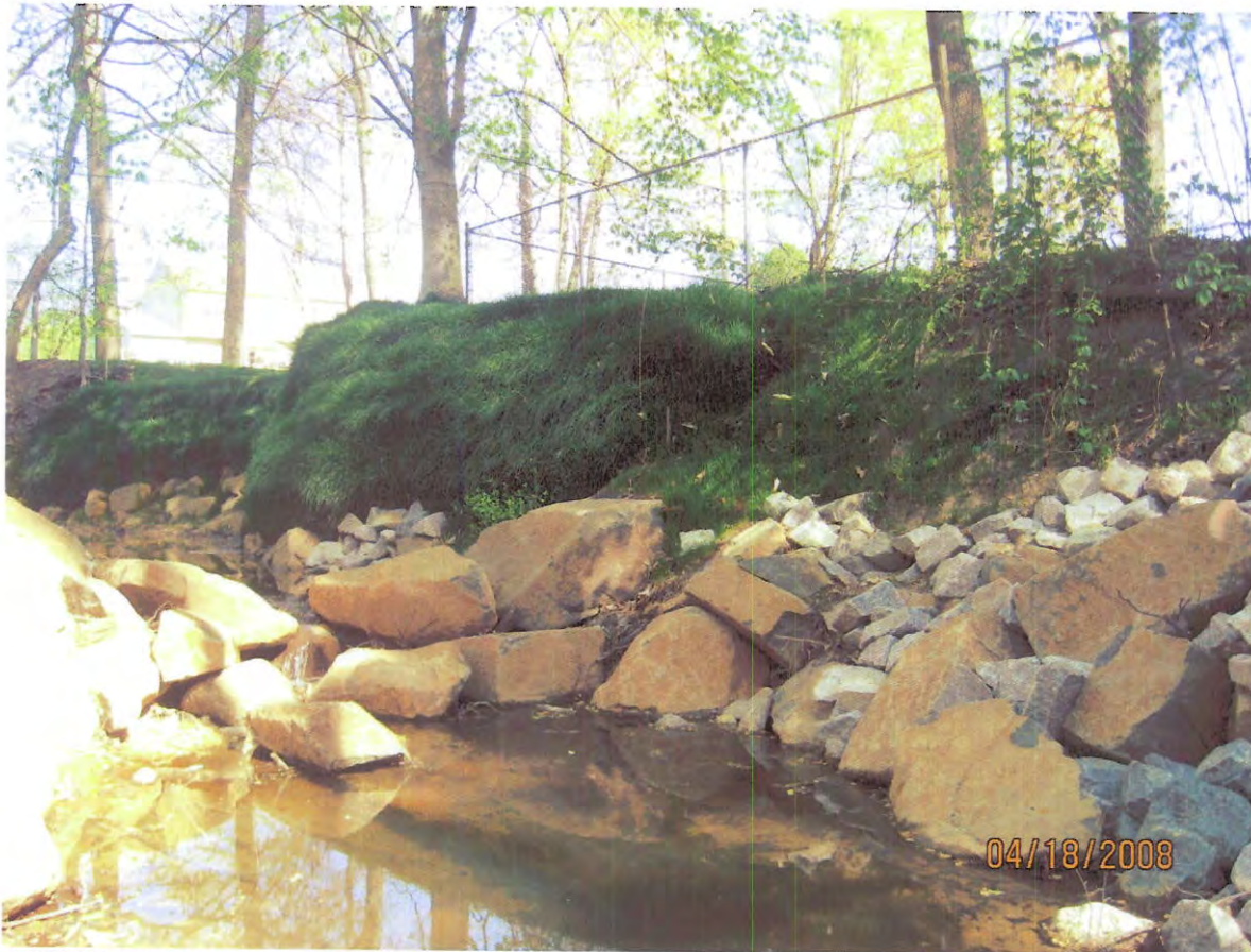
AFTER - Terrace creation and bank stabilization. Near weir #4.
