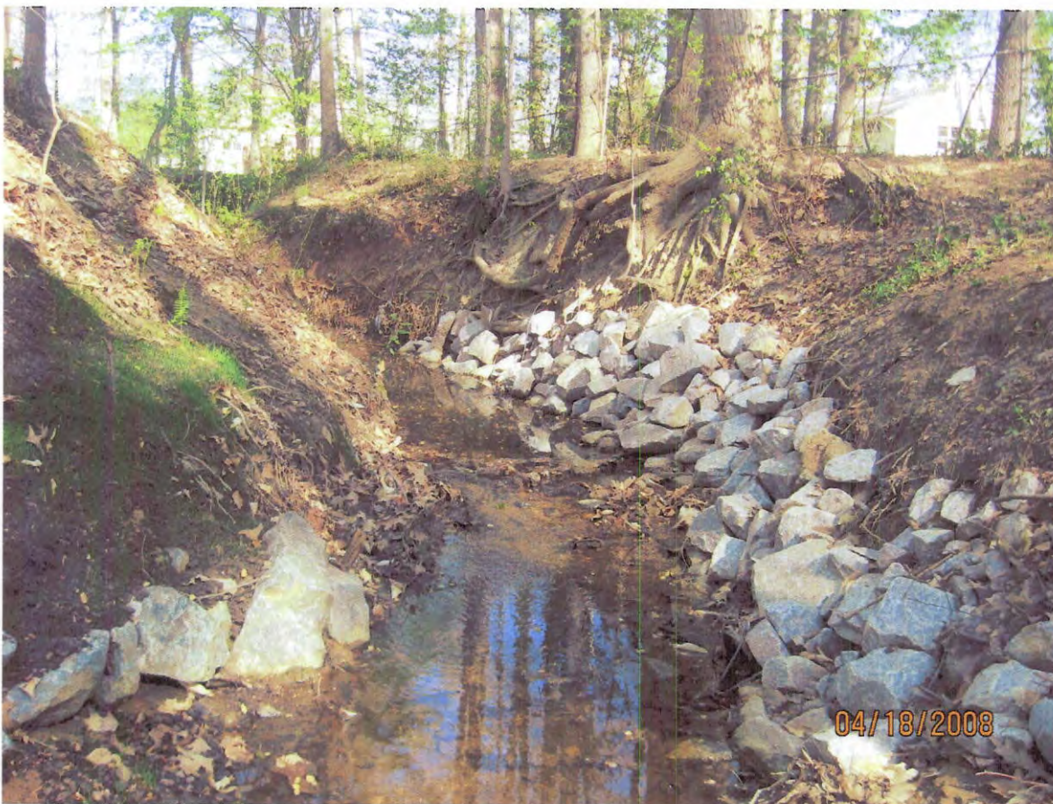
AFTER - bank stabilization upstream from structure 3.
