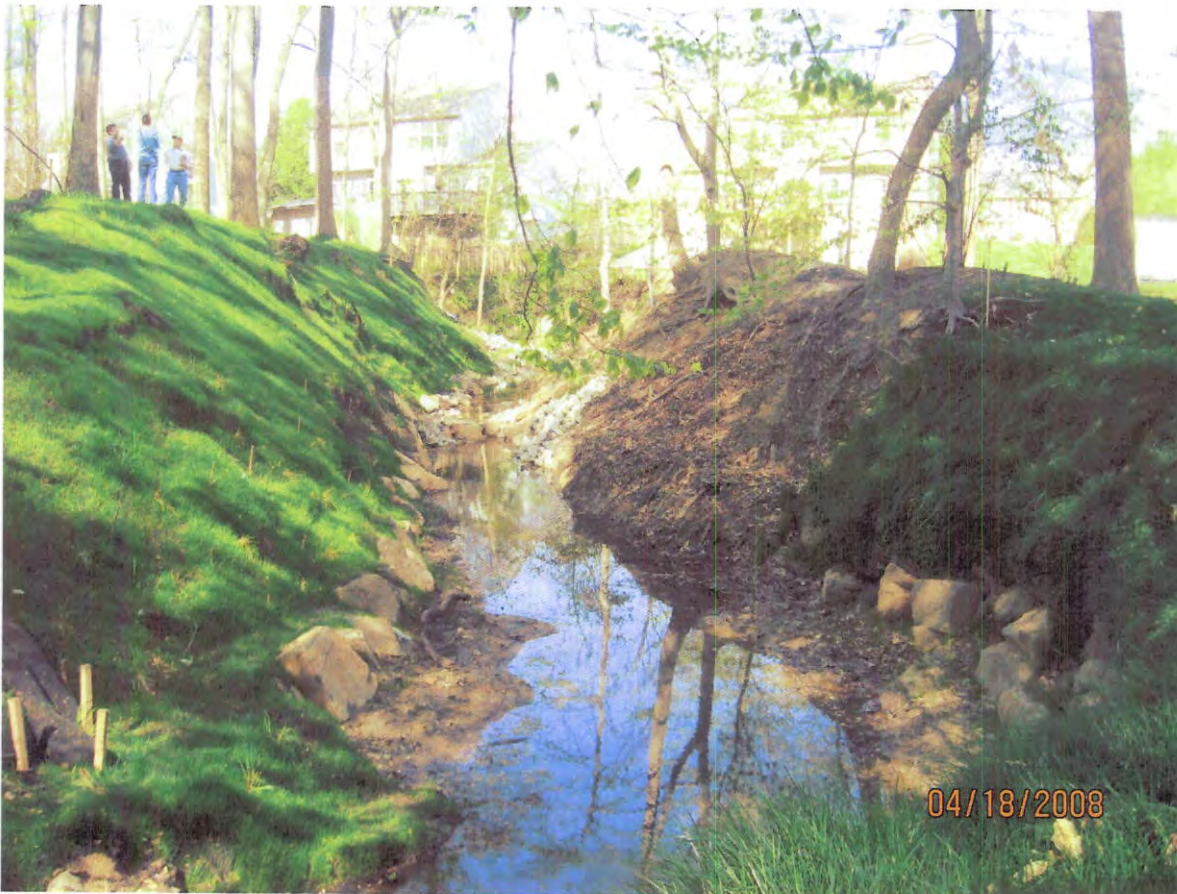
AFTER - stone toe stabilization and bank covered with compost tea.
