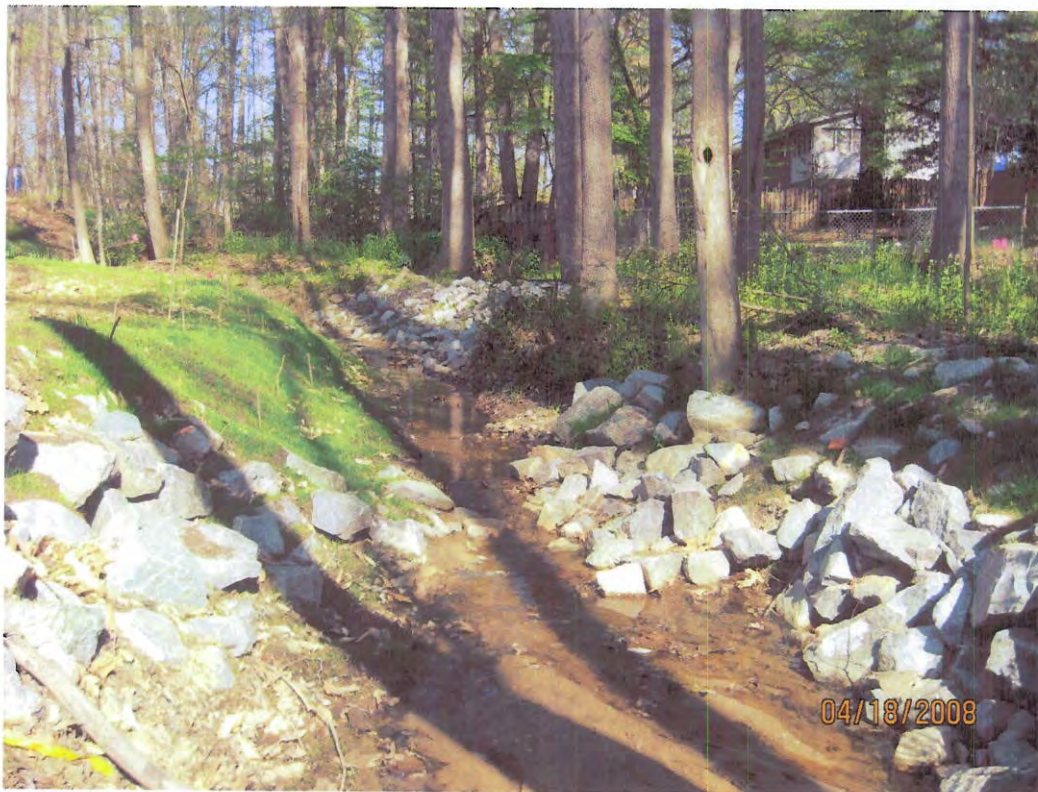
AFTER - Location of #1 rock weir (photo zone 1)
