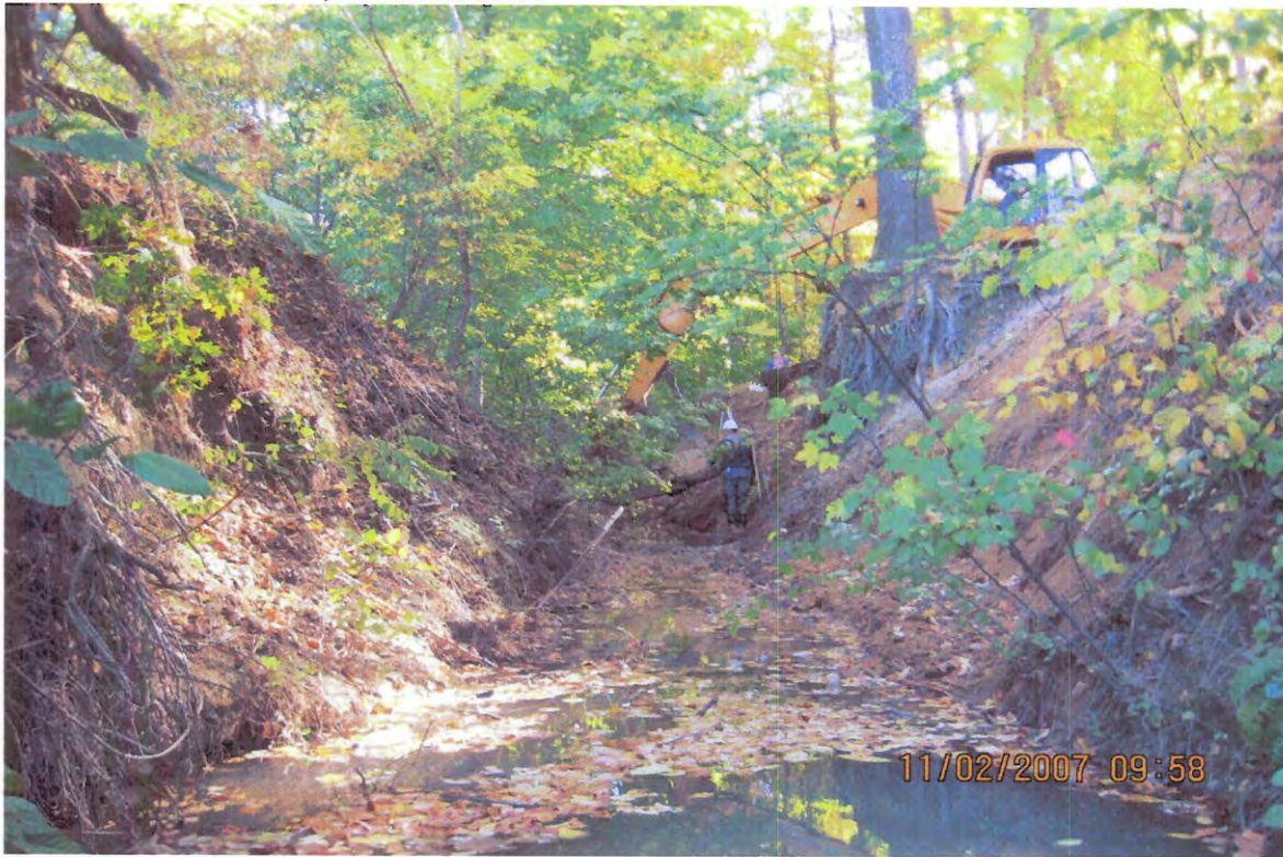
BEFORE – Above weir #5.
