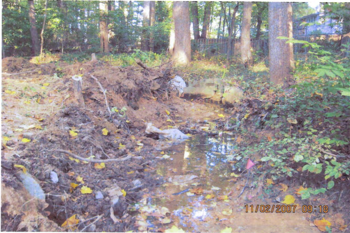
BEFORE - Location of #1 rock weir. (Photo zone 1)
