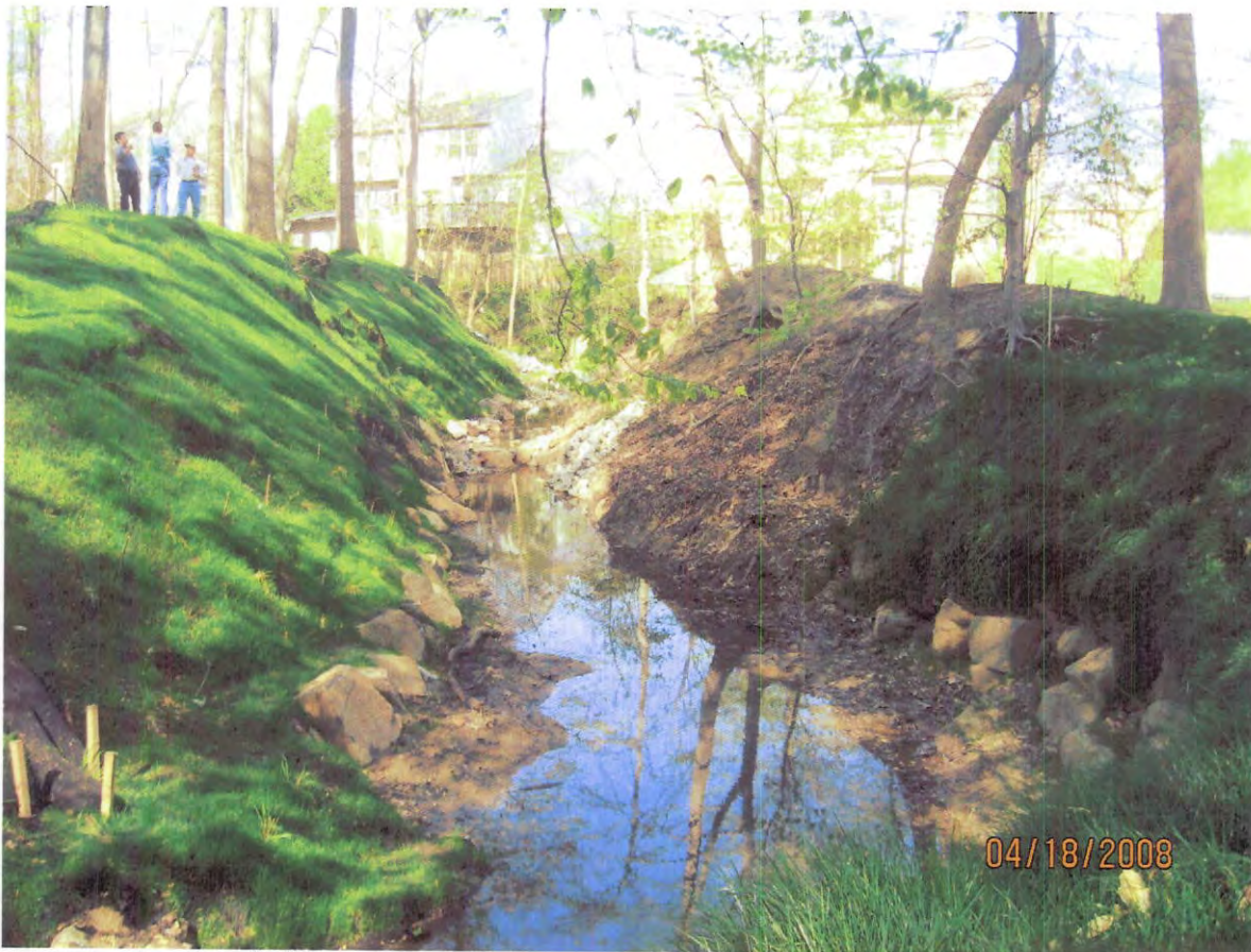
AFTER - Rock weir #5.
