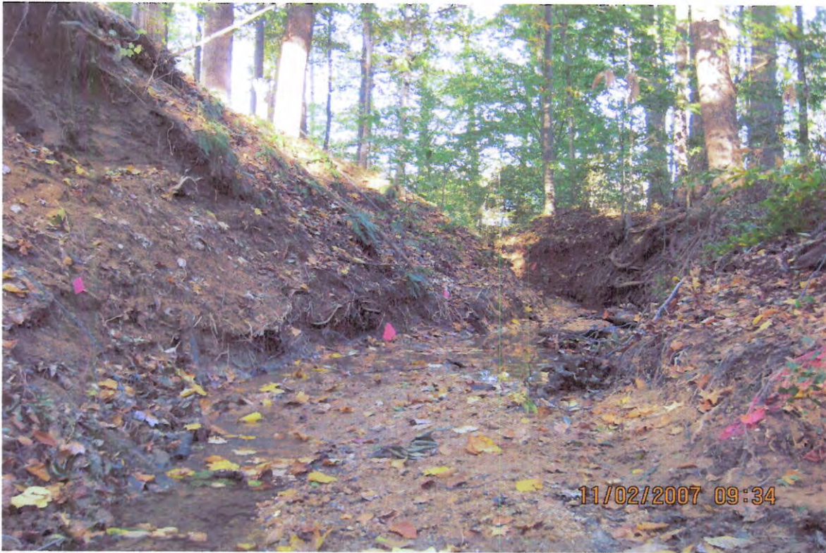
BEFORE - Location for weir #3
