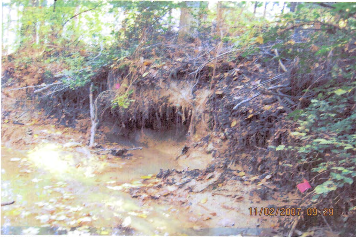
BEFORE – right bank needs rock toe and filtrex sox stabilization.
