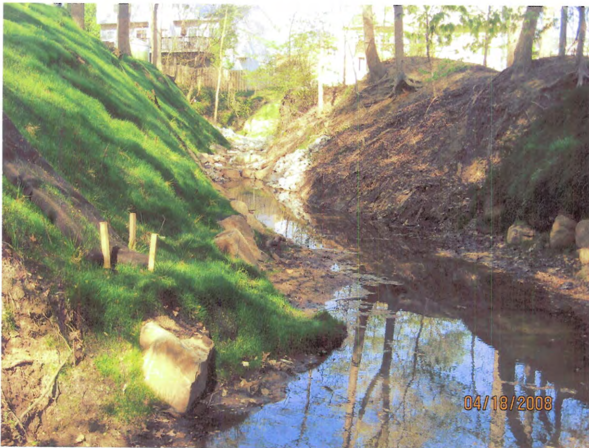
AFTER - Bank cut and stabilization (across from created sill).
