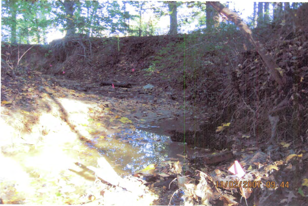
BEFORE - Location to excavate sand deposition bar, create terrace and stabilize bank.
