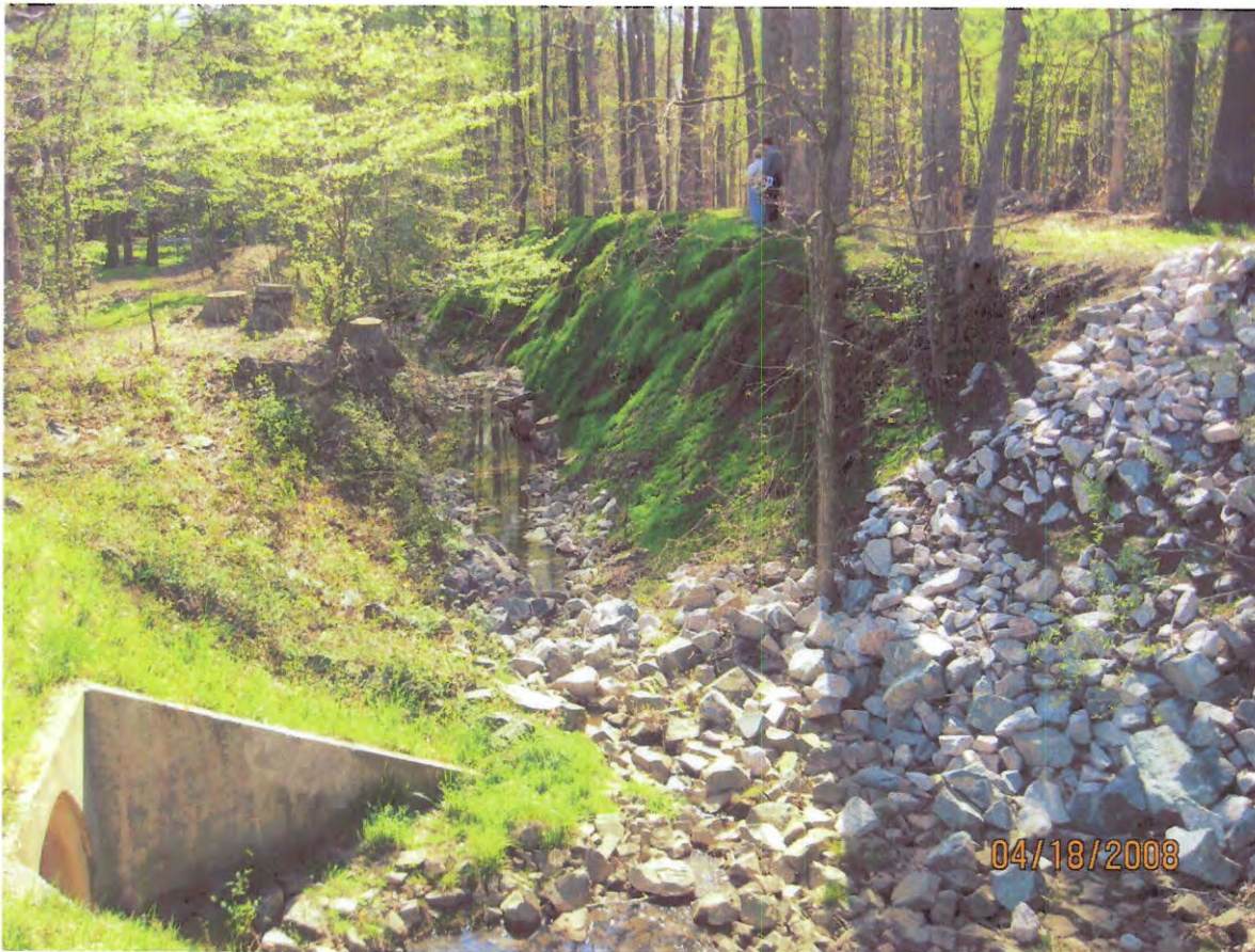
AFTER - At outfall of pond #343, additional placement of rip rap along the slope.
