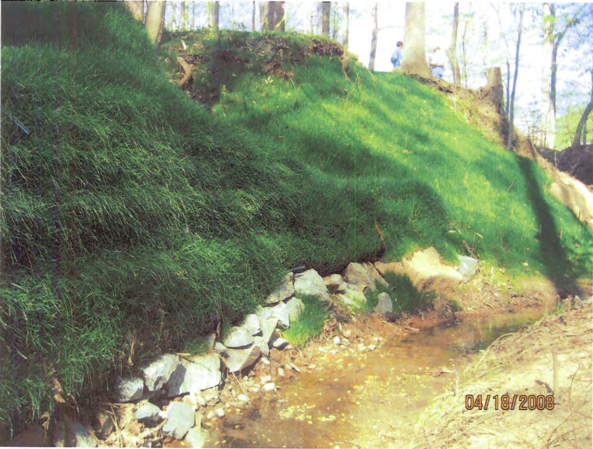
AFTER - Location #8, Terrace slope, filterxx bank stabilization, stone toe.
