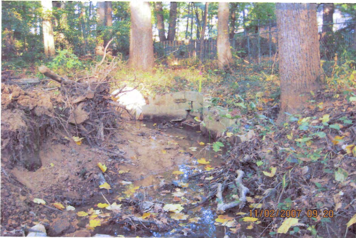
BEFORE - Location #1, need to cut and fill of bank, add stone and mulch treatment to bank .
