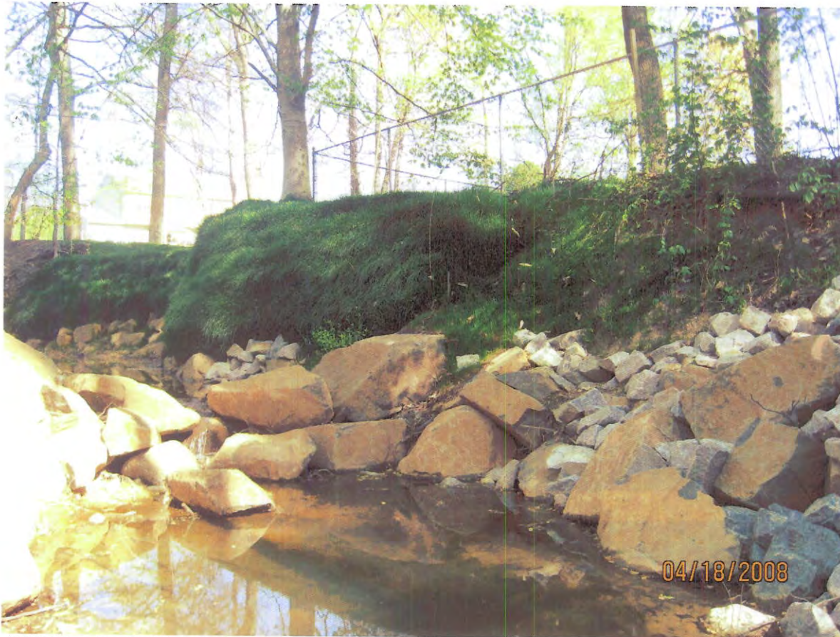
AFTER - Rock Weir #4
