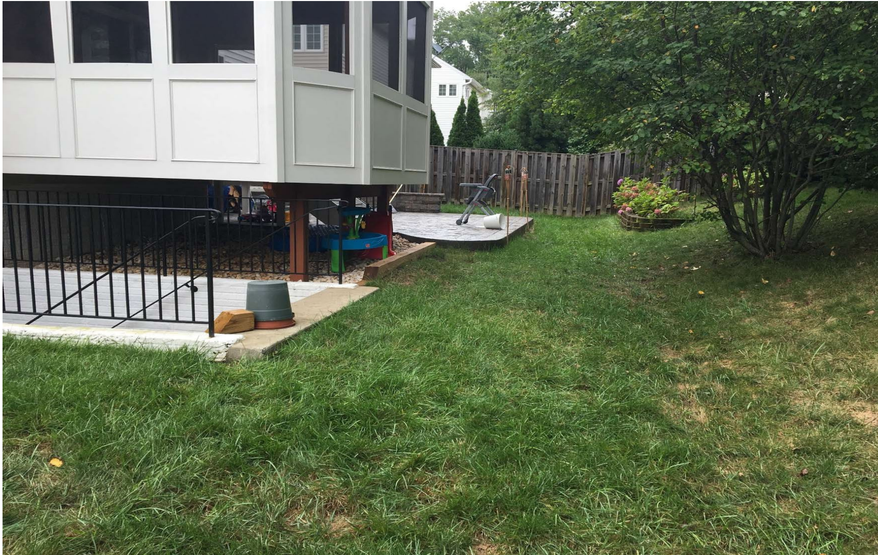
Lack of defined swale directly behind house – note proximity to walk up basement entry
