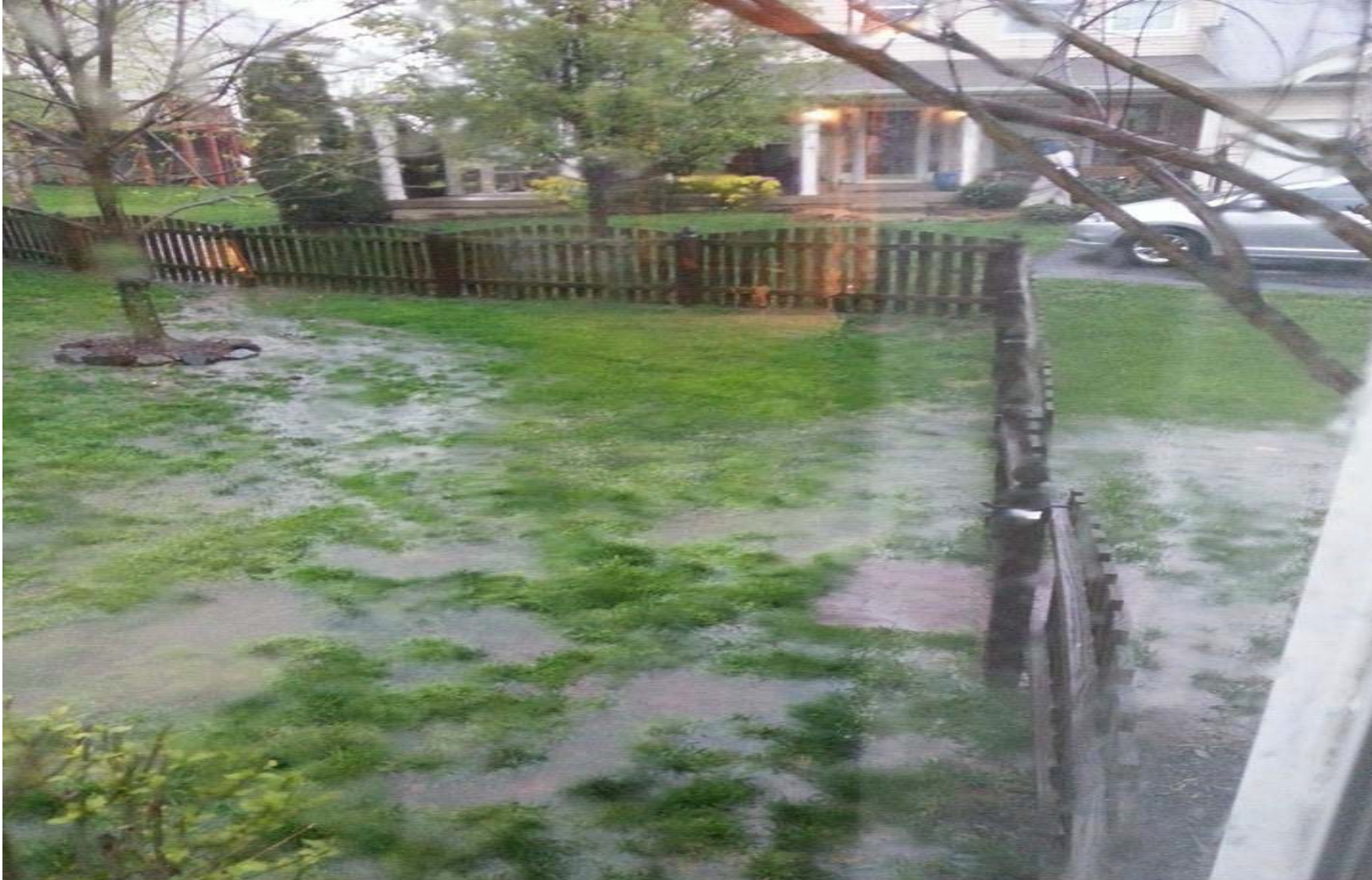
Lack of defined swale causing yard flooding
