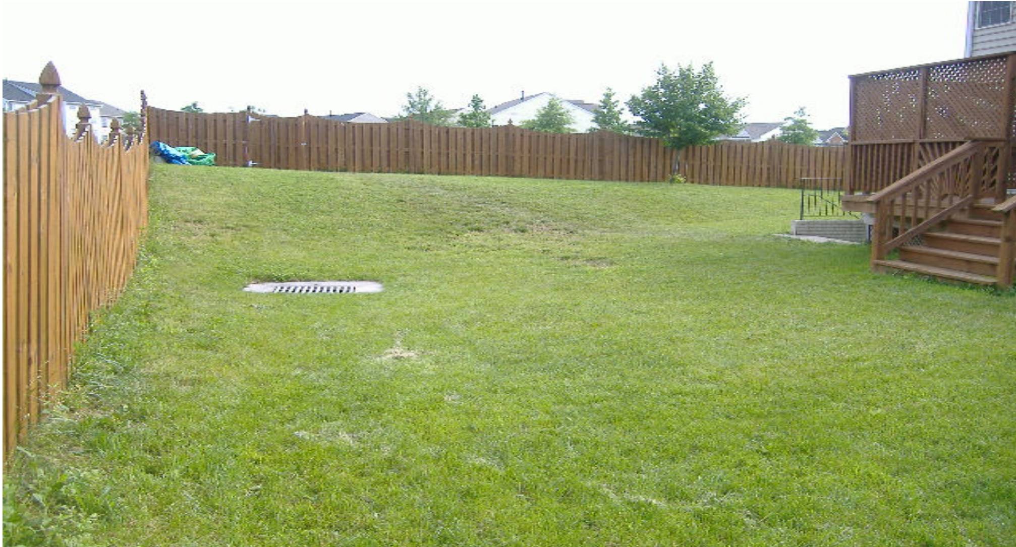
Drop inlet handling large flows close to basement entrance
