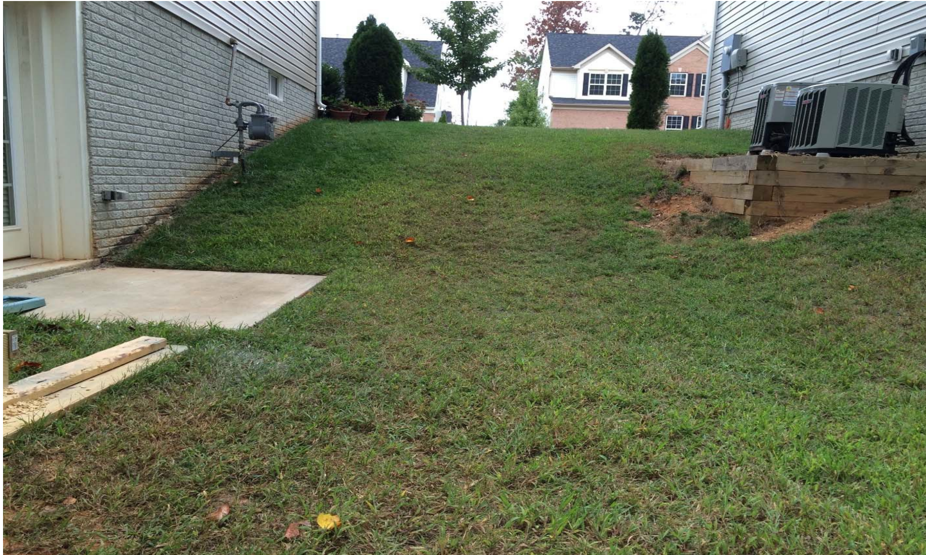
Water directed toward entryway due to lack of defined swale
